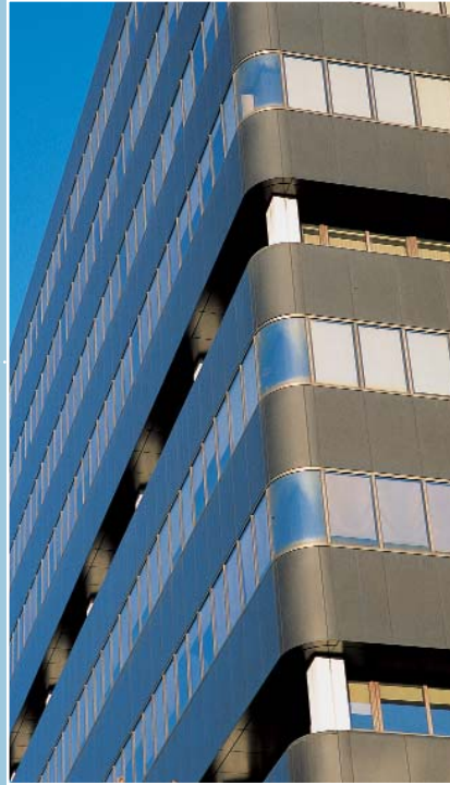
7- MODULAR PANEL SYSTEM FITTED WITH SUB-STRUCTURE AND FITTING GASKETS.
